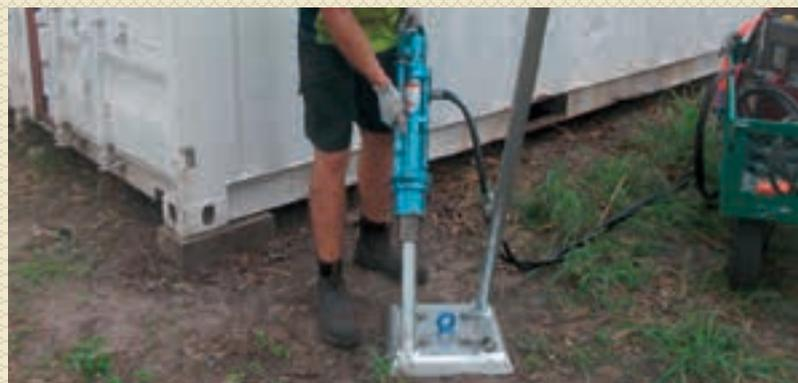
**To remove the pile cap, the micropile should be cut off beneath the pile cap sleeve in order to rotate or relocate the footing**
