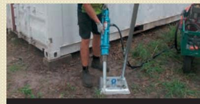
To remove the pile cap, the micropile should be cut off beneath the pile cap sleeve in order to rotate or relocate the footing
